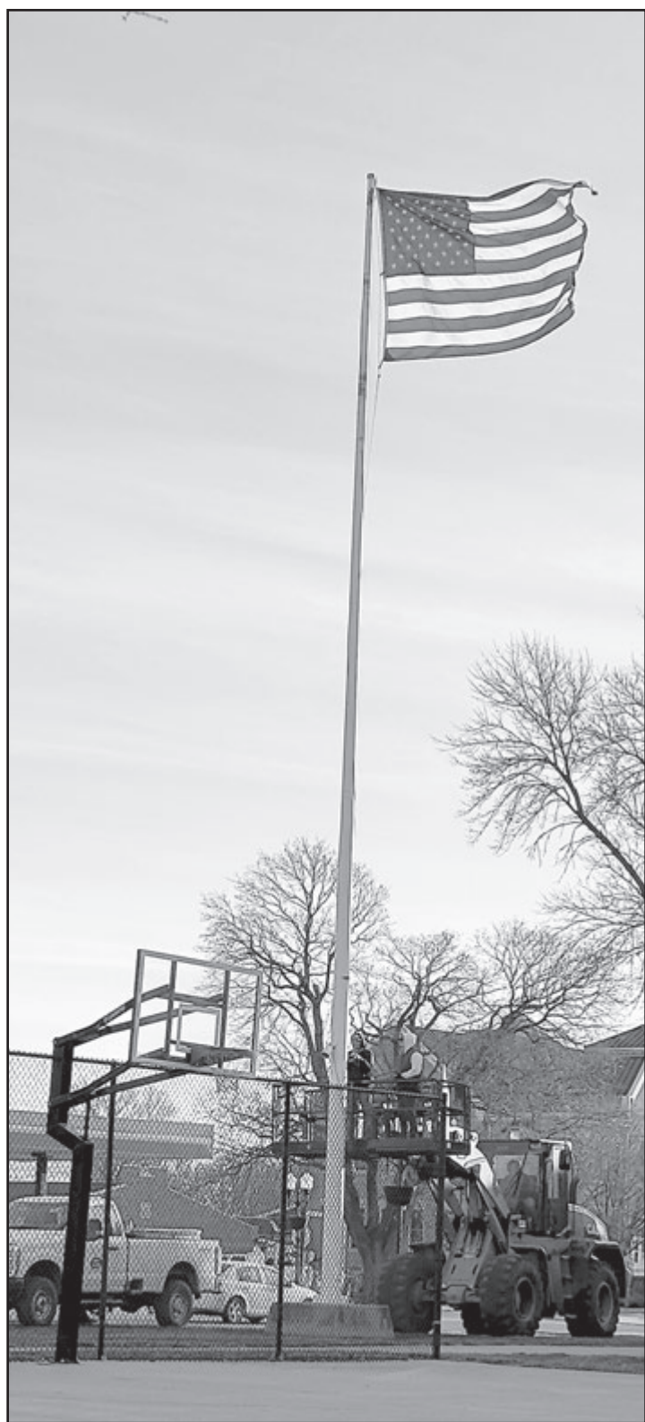
Fixing the flagpole The Northwood public works crew spent some time last week performing maintenance on the flagpole that sits in Central Park, near the basketball courts.
