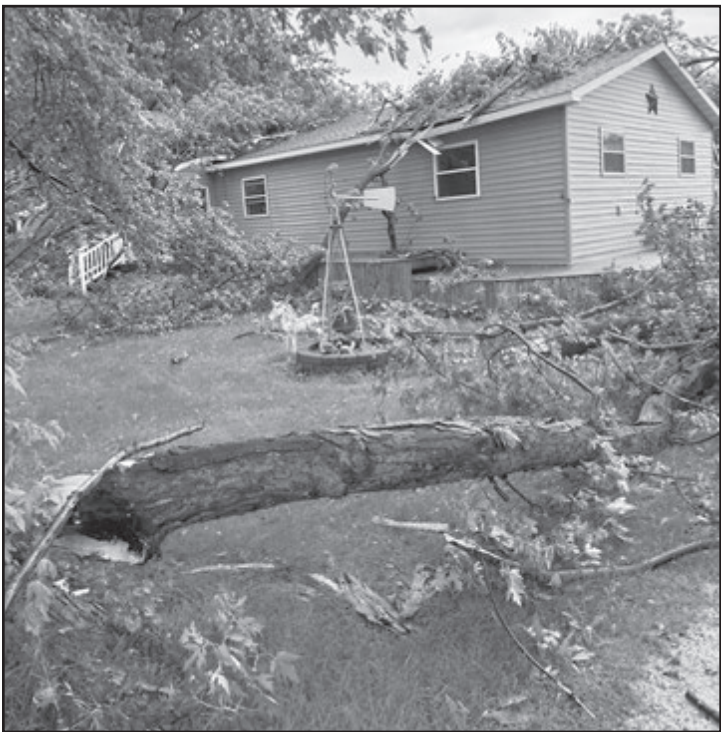
Storm damage Last Thursday’s severe weather brought strong winds through the area. For the Ausborn family of Bolan, that meant substantial damage on their property, with seven trees on their property falling. The trees damaged their roof, shed, septic system, deck, siding and some interior water damage. These images were shared on their Facebook page, along with messages of gratitude for the people that helped and supported them as they cleaned up the aftermath and got ready to rebuild.
